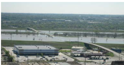
Flooding in Dallas
